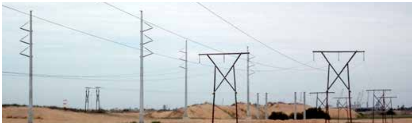
The new Walvis Bay-Kuiseb double 132 kV power line will use steel monopole structures (left) and run parallel to the existing double 66 kV wooden-pole power line (right) (photo credit:Ann Scott).
