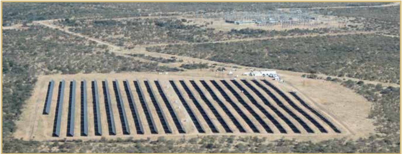
An aerial view of the Omburu solar power plant and the Omburu sub station.
