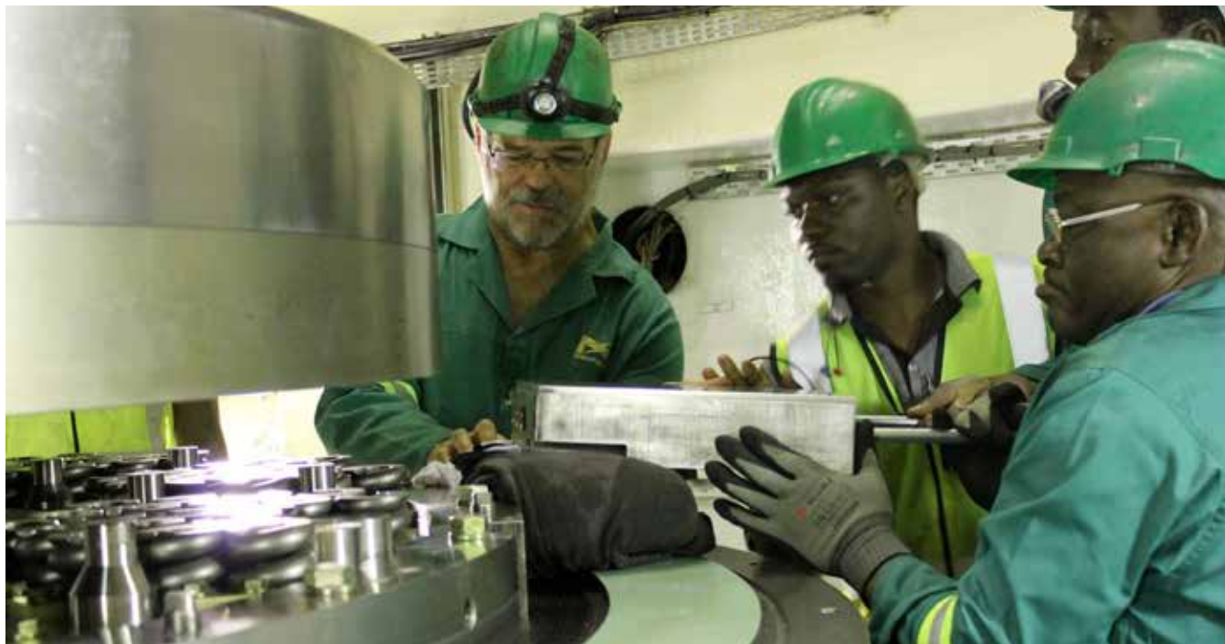
The team at Ruacana installing thrust bearing pads.
